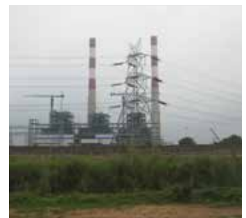
GMR plant under construction in Dhenkanal District, Odisha, India (CAO).
