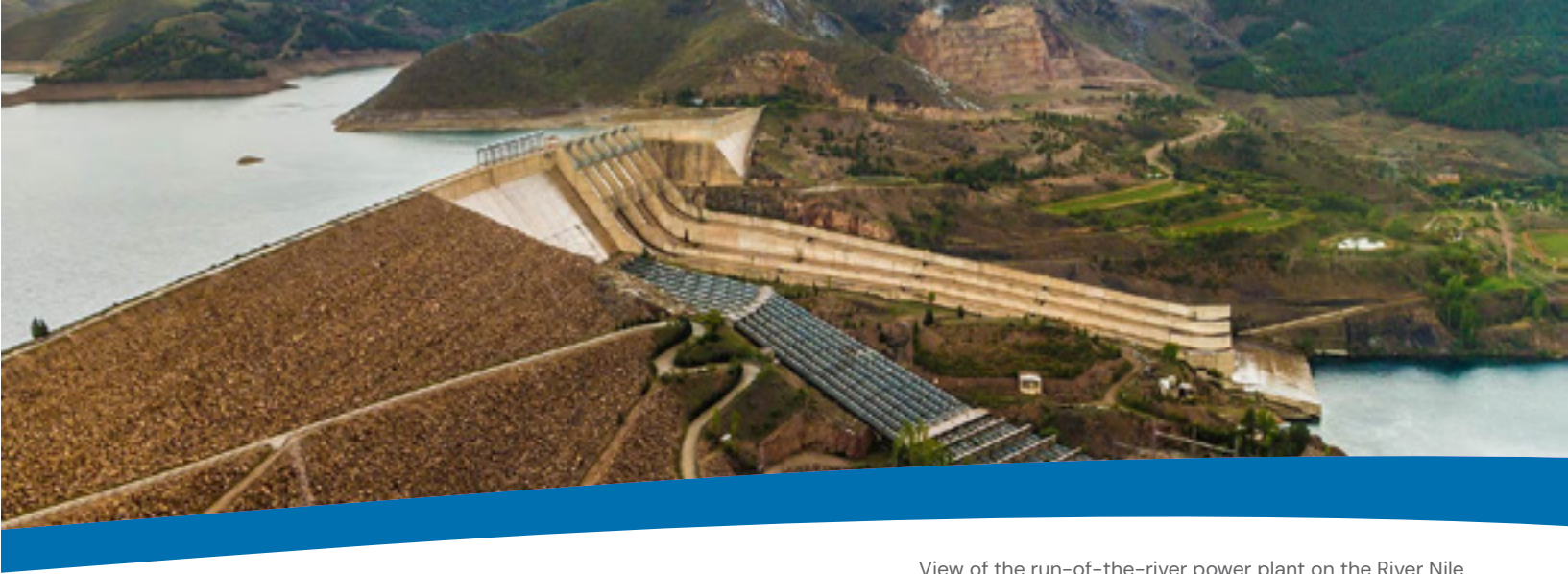
View of the run-of-the-river power plant on the River Nile in Uganda, part of the Bujagali Energy project. (Photo: World Bank Group, 2018)
