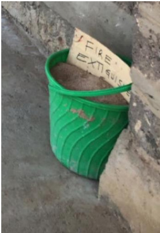
Figure 5. Site photograph of a sand bucket labelled "fire extinguisher," CAO site visit, February 2020.
