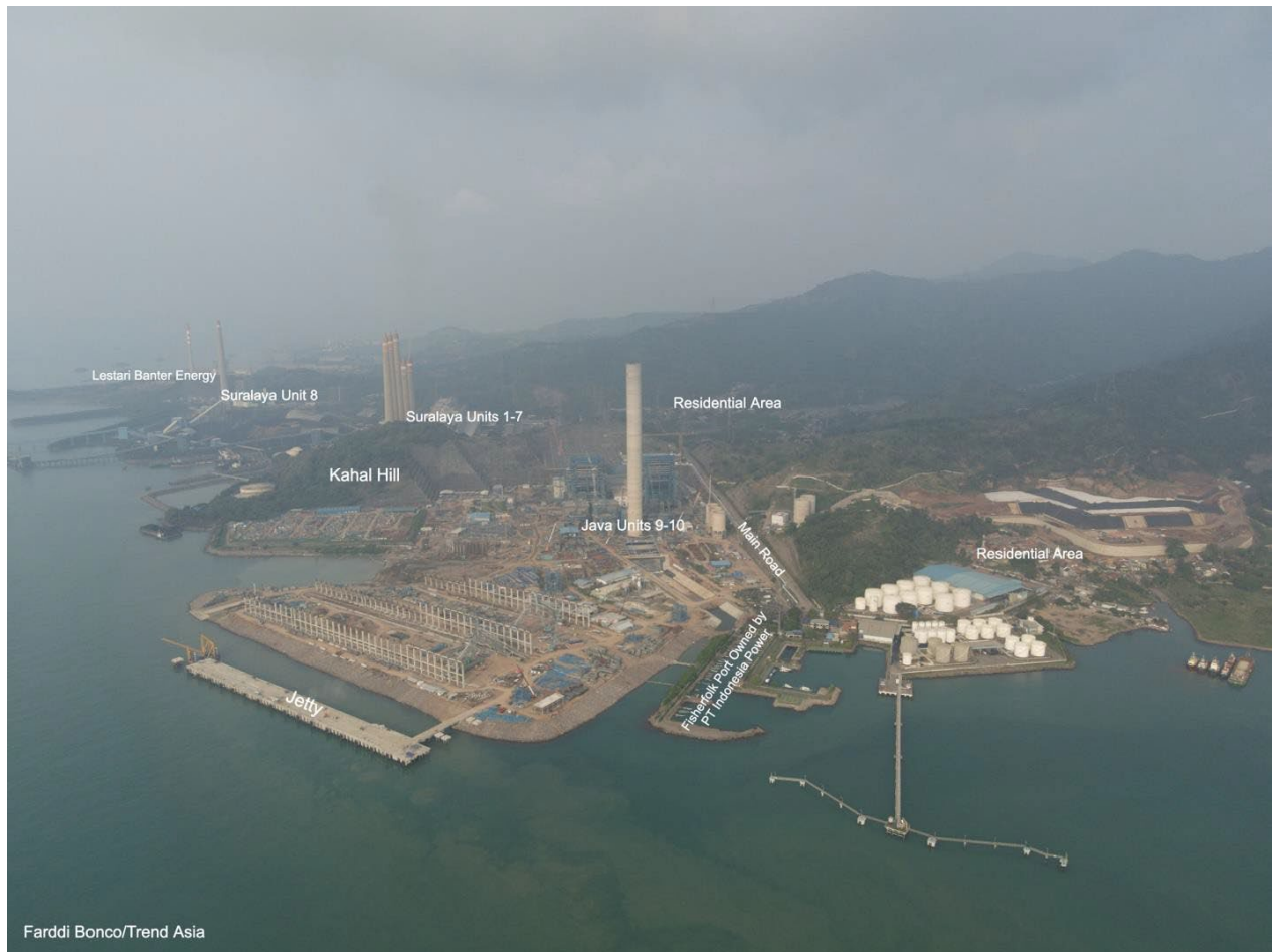
Partial construction of Java 9 and 10 (July 2023).
