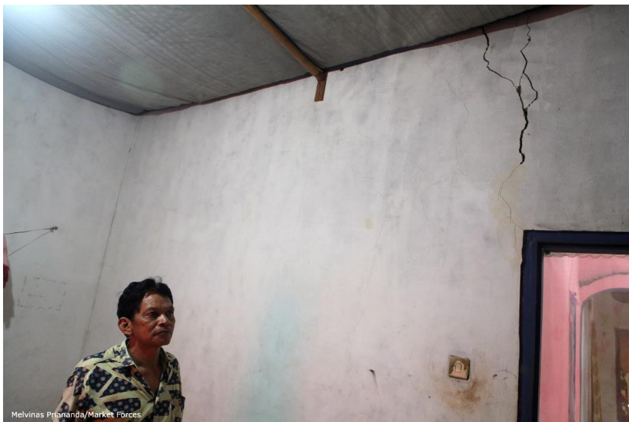
Blasting damage that occurred in 2017 at the start of Java 9 and 10 construction (2021).
