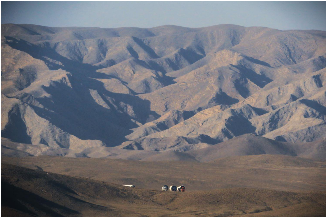
Construction of wind turbines with Mount Aktau in the background. CEE Bankwatch Network, February 2024
