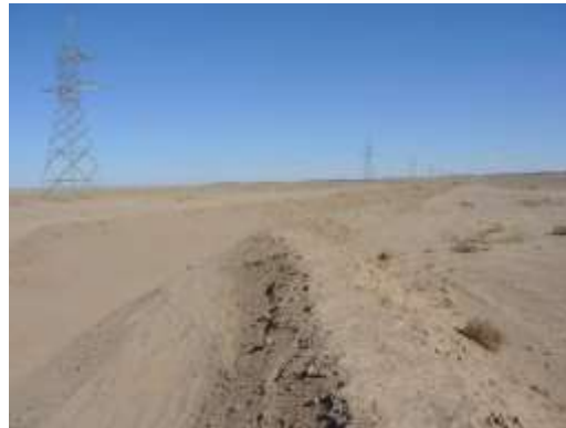
Diversion ditches in Haliv Dugat area, north of Tailing Storage Facility.
