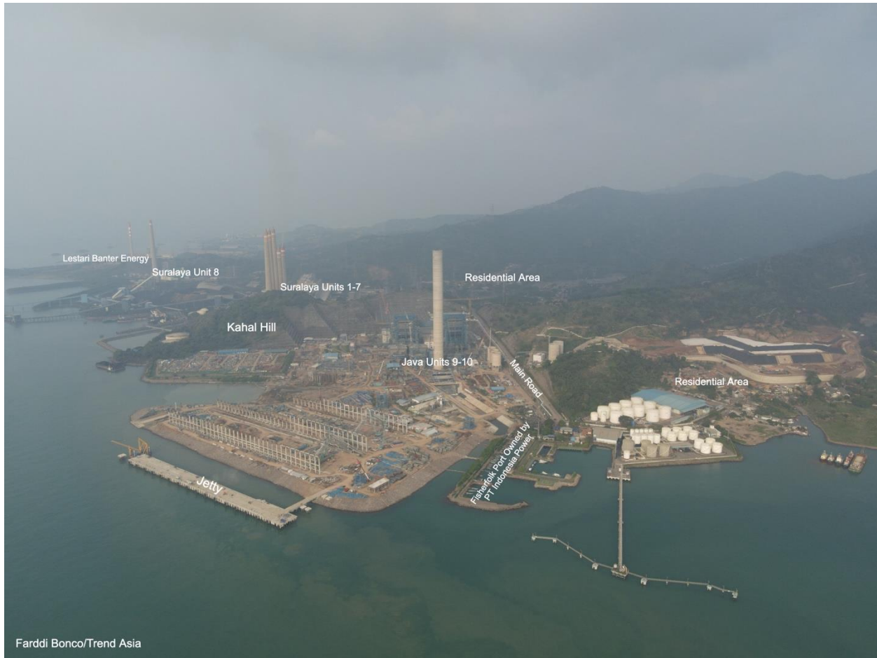
Partial construction of Java 9 and 10 (July 2023).
