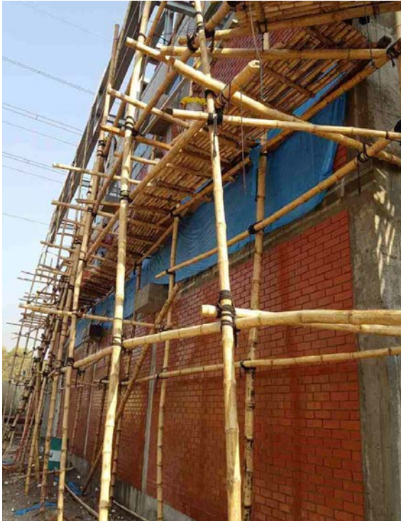
Noise-reduction measure in progress
